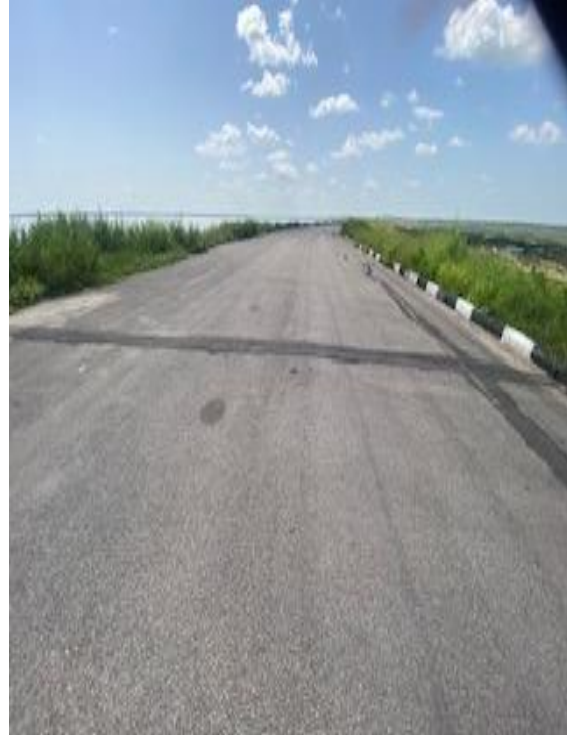
Figure 8: A section of the Dam Crest
