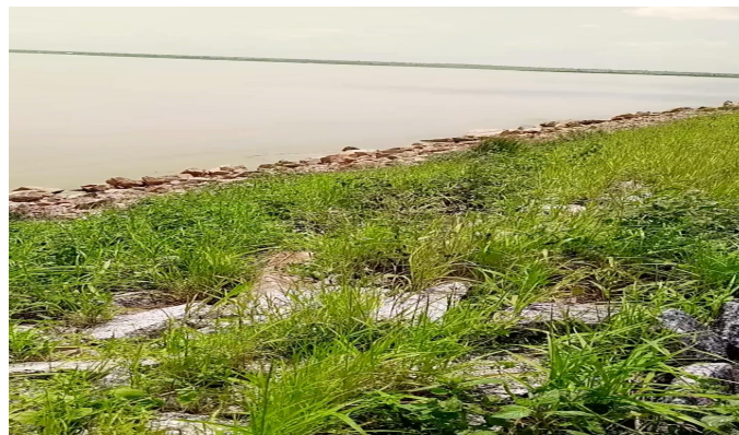
Figure 5: Upstream Slope protected with Riprap
